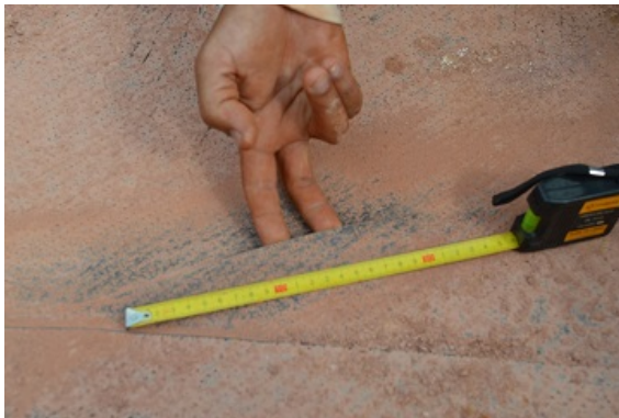
Figure 5. Cut damage.
