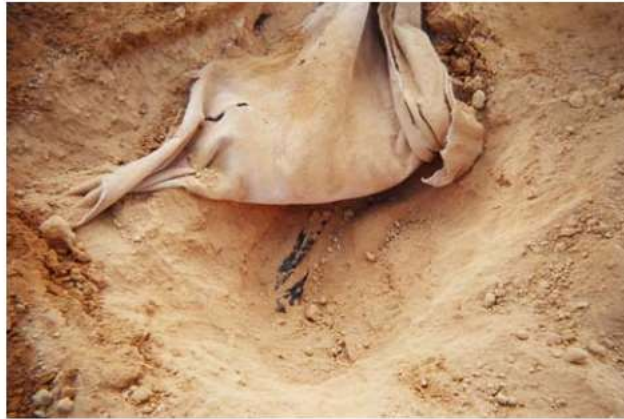
Figure 5. A one meter tear discovered using the dipole method, caused by heavy equipment during covering material placement.
