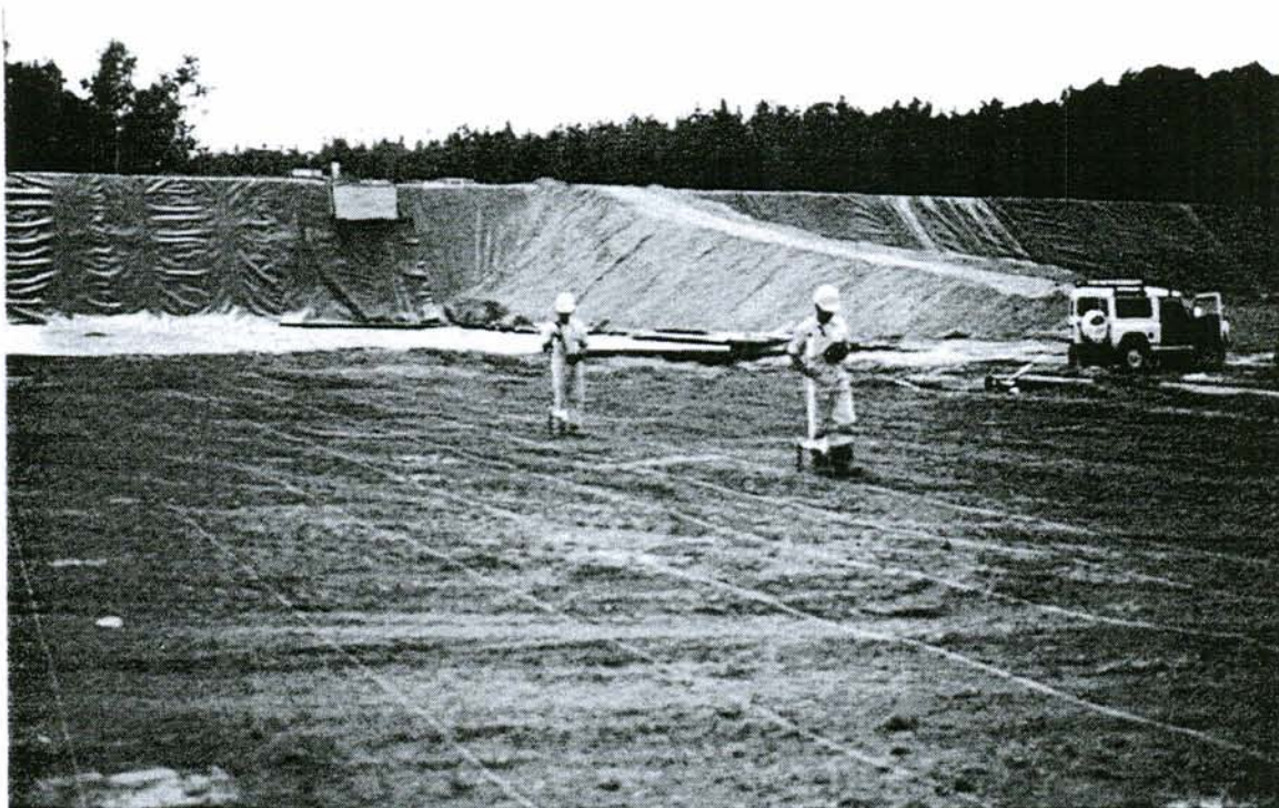
FIGURE 3. LEAK LOCATION SURVEY WITH SOIL COVER
