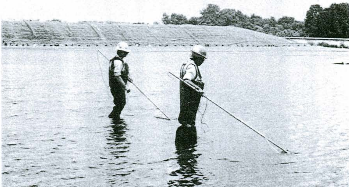
FIGURE 1. LEAK LOCATION SURVEY WITH WATER COVERING THE LINER
